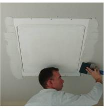
1. Apply drywall mud base, covering seems and screws.
