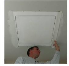
2. Apply drywall tape, also covering seems and screws.
