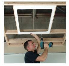
2. Affix panel frame by screwing it into ceiling frame using pre-marked divots.
